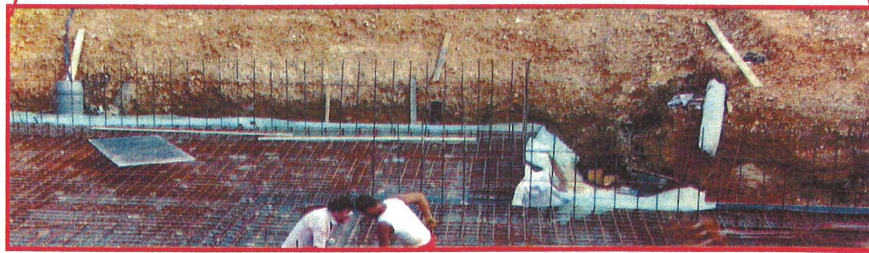
Blown up to show vertical reinforcing bars of continuous garage and house walls fixed to single garage and house foundation slab.
